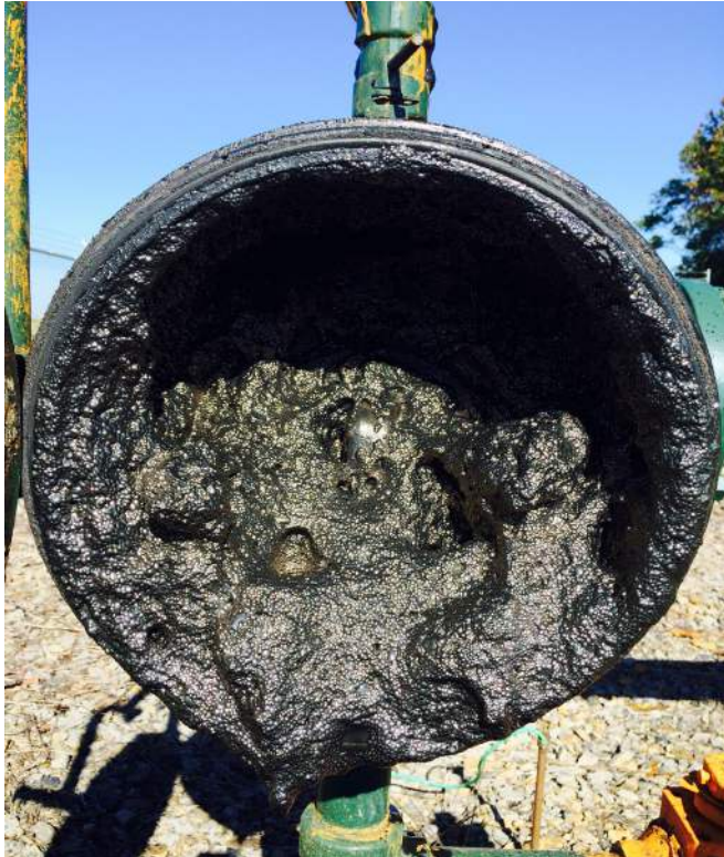
Figure 1. An extreme case of iron sulphide or better known as black powder, build up inside of a pipeline.
